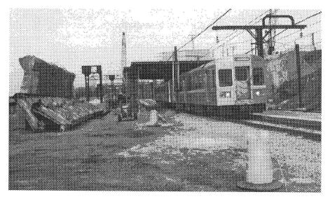
In early January the contractor began removing the 34th Street structure in Cleveland. My firm has a contract with NS to observe the demolition of the bridge that was constructed in 1920. In this photo the bridge is gone. Two of the 80 foot girders lay against the pier on the left. The rapid transit has just left Terminal Tower and is eastbound by the site. Photo by Rick Schroeder
