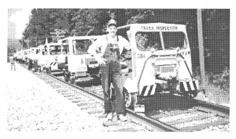
In the photo we are stopped at Milepost 209.8, the Seiver passing track, holding the mainline on the southbound leg of the trip. The motorcar is a Fairmount M-19, a former C&NW car.
