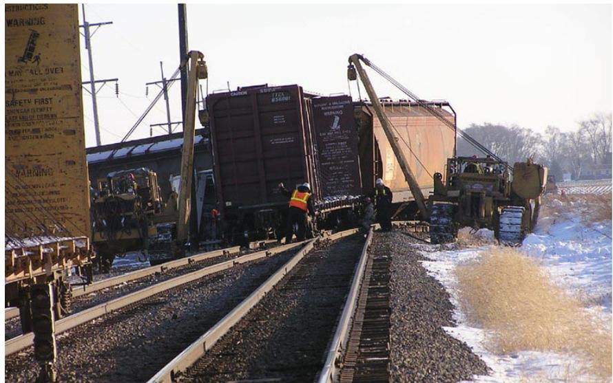
Hulcher is in the process of setting a car back on the track at Wellington. The switch, signal equipment and several hundred feet of track were torn up as the southbound was departing the siding. *Photo by Joe Cooke.*
